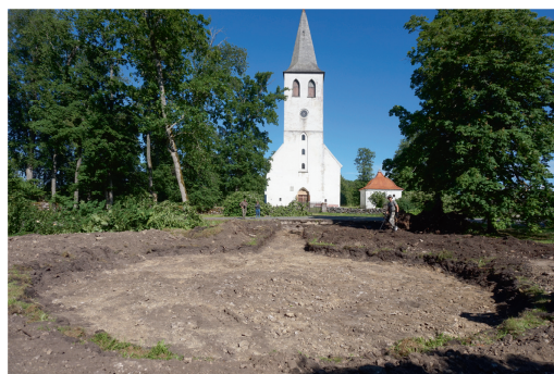
Fig. 3. The foundation pit of the monument after archaeological research.
