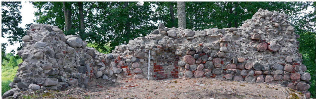
Fig. 4. A room in the northwest part of the castle, in which remains of brick vault arches and a brick-lined niche were discovered.
