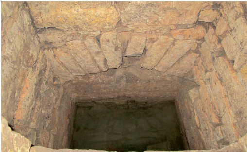
Fig. 6. The current water level in the well that has been hewn into the natural limestone is 1.2 m above sea level, yet before the moats were dug for the castle-fortress, water level extended to a considerably higher elevation. A relieving arch is visible in the wall of the well.
