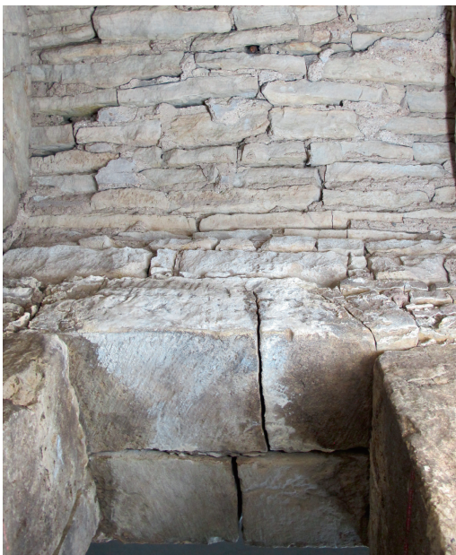
Fig. 7. An iron rod was bricked into the well's ceiling. A bucket hung from a rope tied to that rod. Traces of the rope worn into the doorjamb indicate that the well was used intensively in the Middle Ages.
