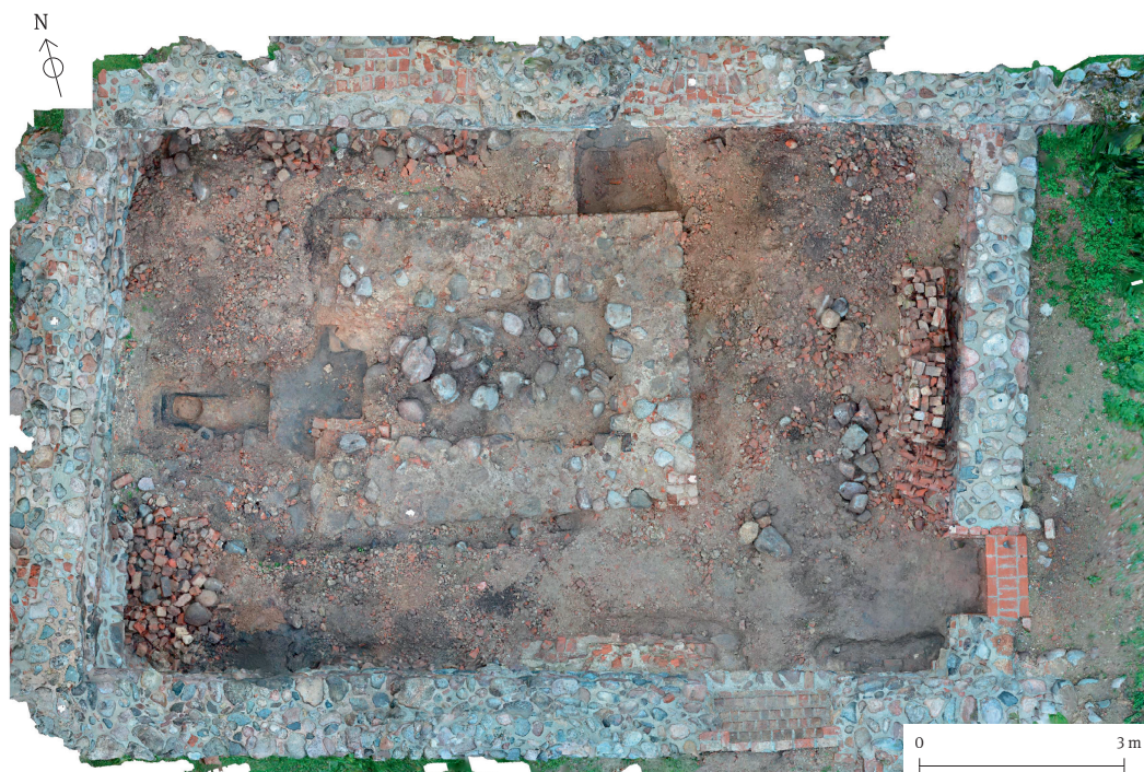
Fig. 8. The western room of the 'Clergy house' in Viljandi with discovered walls of an unknown building.
