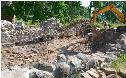
Fig. 3. Removal of debris from the western room of the ‘Clergy house’.
