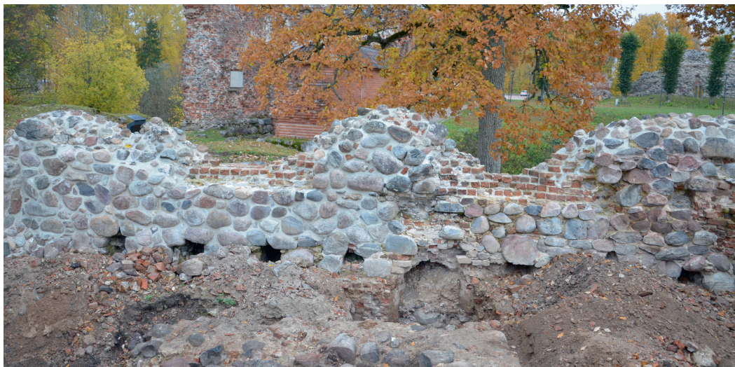
Fig. 10. Openings for beams in the northern wall of the 'Clergy house'.
