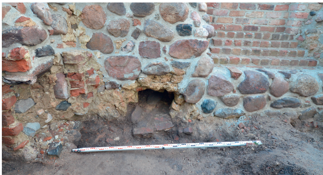
Fig. 11. An opening of unknown purpose and vault-basis like construction in the south-eastern corner of the room (after conservation).
