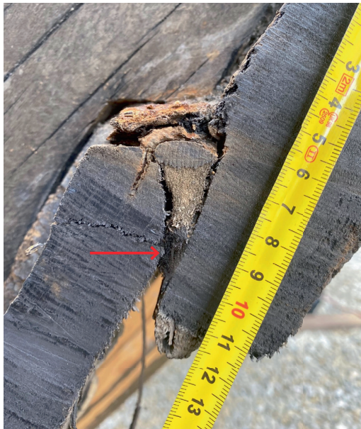
Fig. 4. Caulking between two planks. Animal hair marked with the red arrow.
