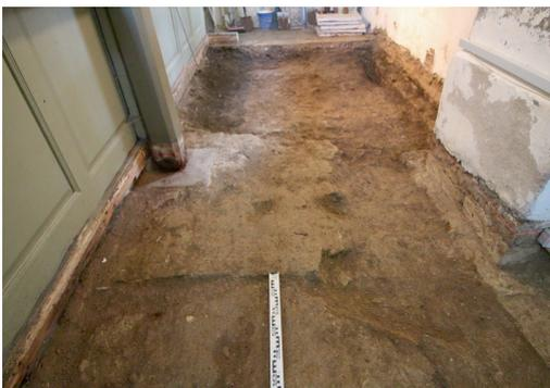
**Fig. 5.** The foundation of the southern wall of the old nave between the nave and the southern range.
