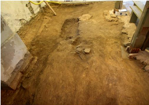
**Fig. 4.** Hardened soil of the late medieval floor in the south-western part of the nave. Foundation of the southern wall of the nave (left above), single grave, foundations of a previous gallery posts (middle), existing gallery posts with a square floor slab for foundation (right).
